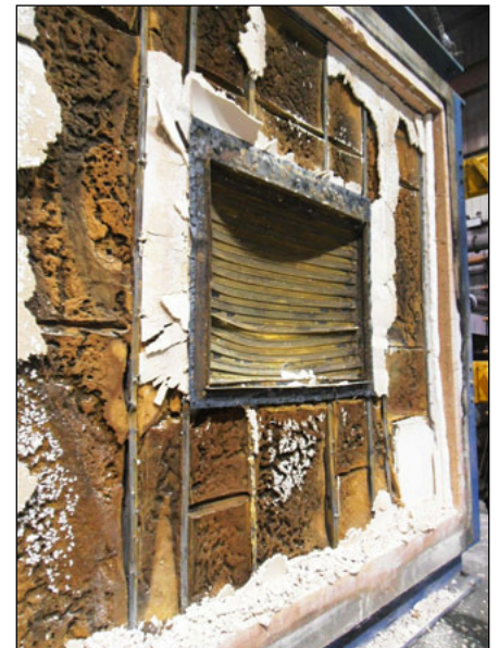
Fire damper and the remains of a drywall partition after a fire test.
